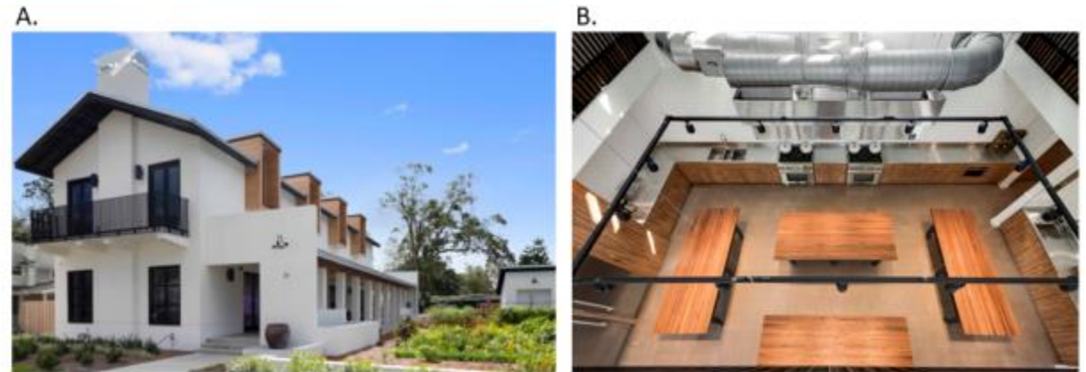
Figure 2. The Emeril Lagasse Foundation Kitchen House and Culinary Garden in Orlando, Florida: (A) exterior (veranda) and (B) aerial view of interior.
